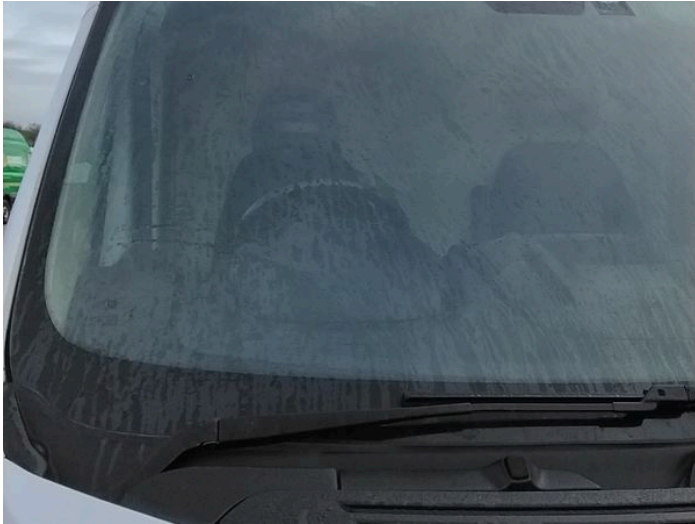
1: Screen Front Chipped Over 10mm
